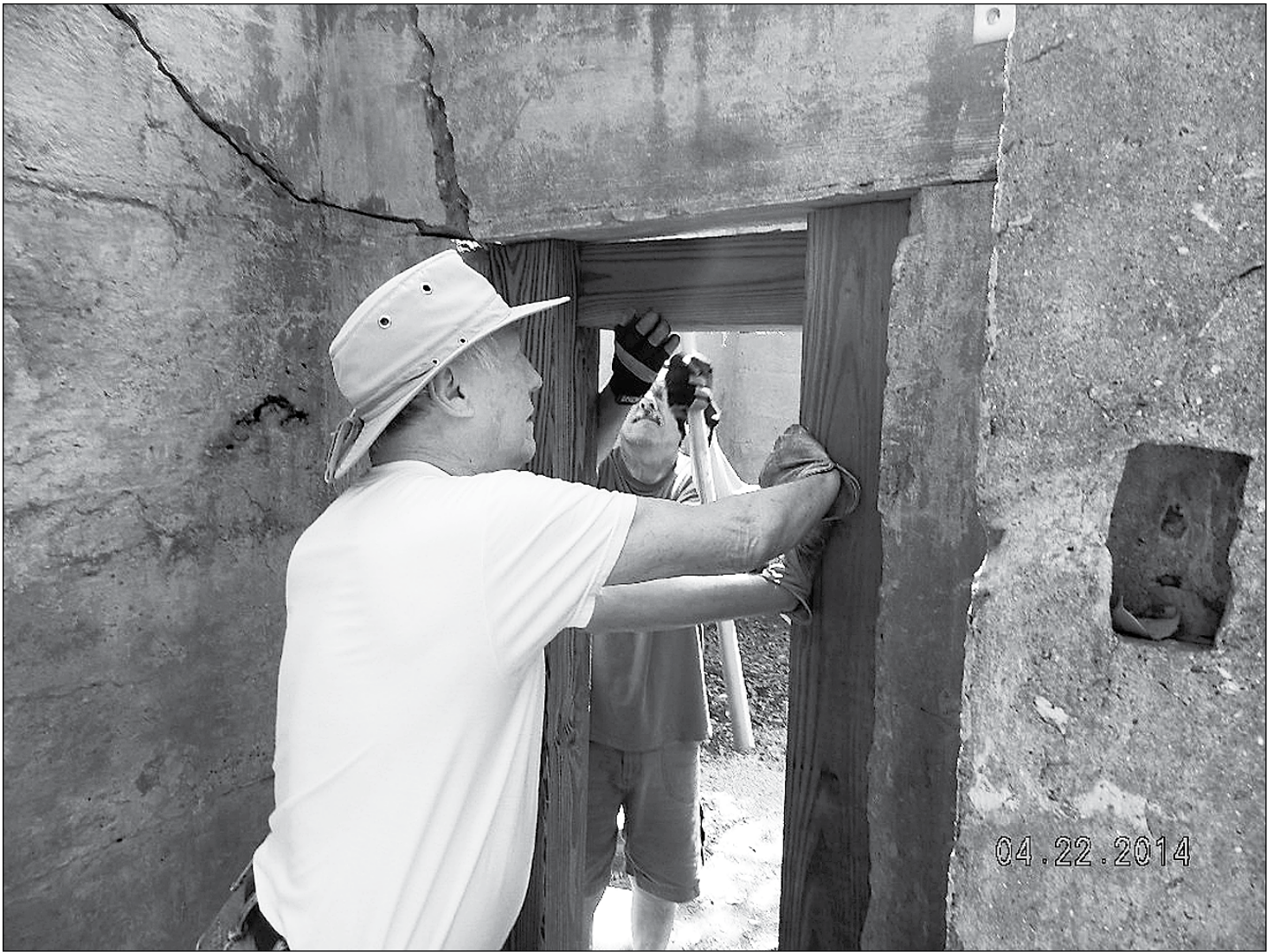
Photo supplied Joe Higginbotham (foreground) and Victor Cash install supports to brace and stabilize the lintels of the World War I-era rifle range pit at Caswell Dunes. The structure is among the few remaining examples of how Americans trained before being sent overseas.
