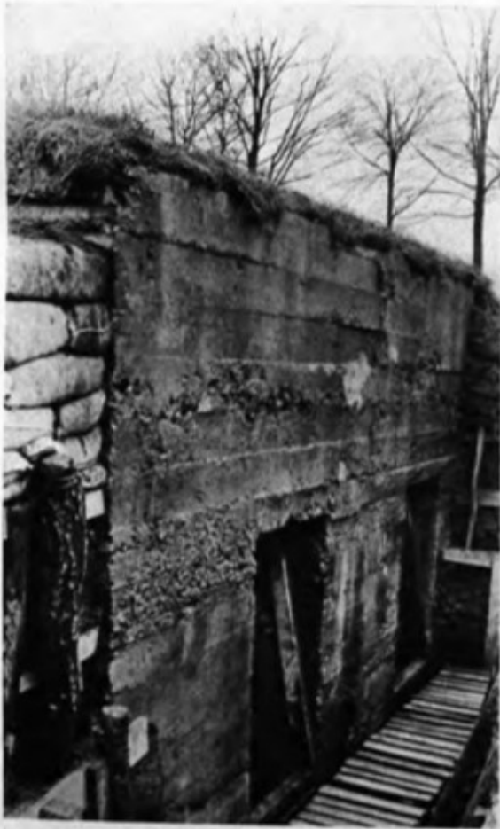
30. A MONOLITHIC CONCRETE MACHINE-GUN PILL-BOX, CANAL SECTOR, BELGIUM Built by the 105th Engineers
